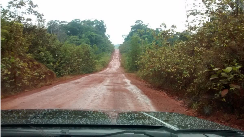
Figure 7: Unpaved stretch of BR-156 (towards Oiapoque/Macapá in January 2020)
