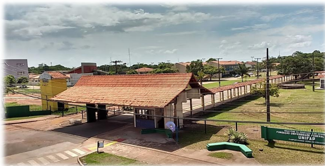
Figura 9 – Entrada principal do Campus Marco Zero
